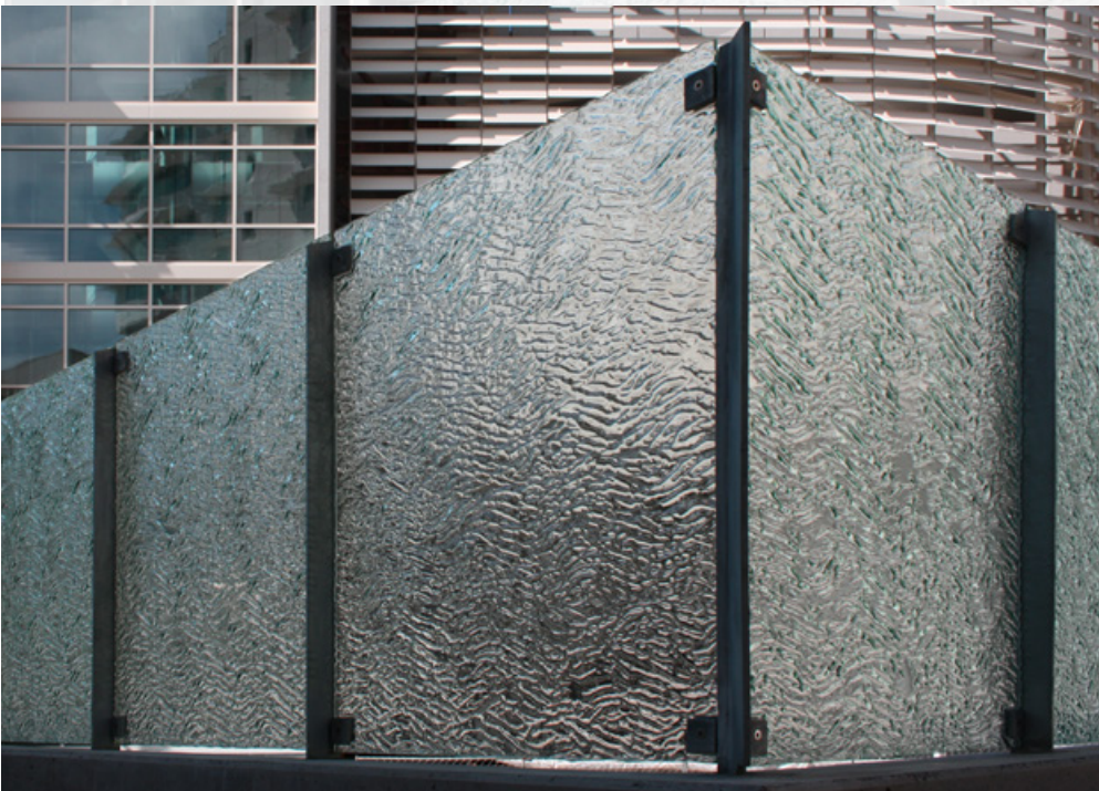
UC DAVIS MEDICAL CENTER - SACRAMENTO, CA - Kiln-Fired Tempered Glass for Exterior Wind Screen - Shown in Horizontal MD202 Flow 1/2" Clear
