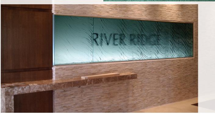
RIVER RIDGE - FORT LEE, NJ - Kiln-Fired Tempered Glass for Interior Feature Wall / Signage - Shown in MD211 Splash in 3/8" Blue Green Tinted Glass Kiln-Fired Glass for Art & Architecture
