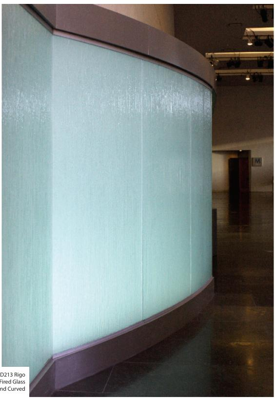
Texture: MD213 Rigo 1/2" Starphire Tempered Kiln-Fired Glass Frosted and Curved
