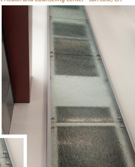
Texture: MD231 Anime 1/2" Clear Tempered Kiln-Fired Glass 60 Minute Fire-Rated Transparent Wall
